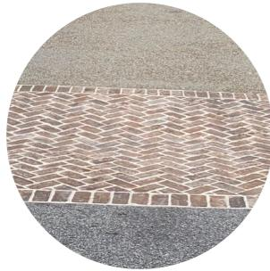
Some pavers themselves are pervious and some are not, but if installed correctly, they will all allow water to penetrate in between each paver.
