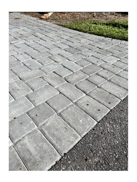
If you are replacing or building a driveway, patio, or walkway consider a pervious material to allow water to penetrate through the surface and absorb into the ground.
